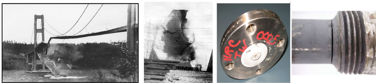
Figure 3-7 Suspension bridges, cooling towers, and thermowells adversely impacted by wake frequency
