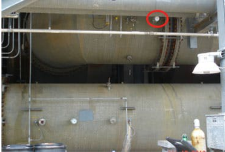
Typical thermowell installation on outside elbow of circulating water line.
